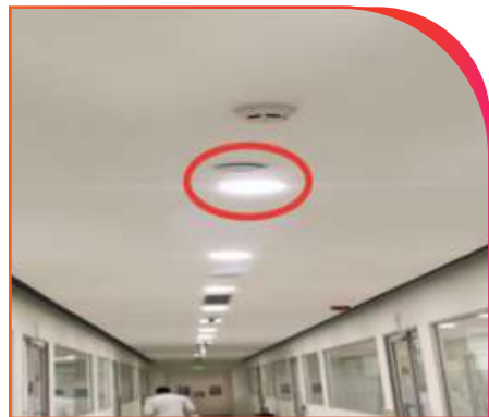
Installation of Motion Sensors
