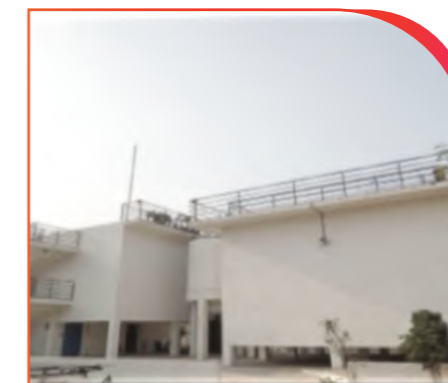
Effluent pre-treatment facility @MLR
